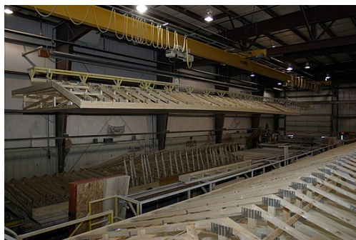
Roof assembly is set atop home.
