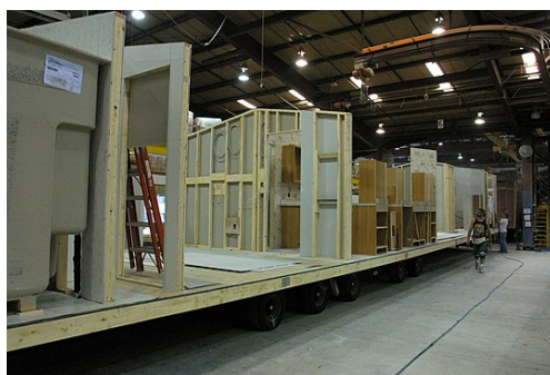
Interior wall assemblies are attached.
