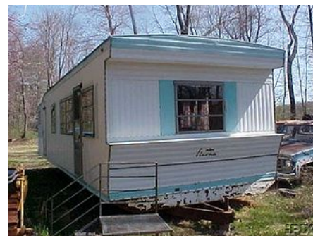
Typical mobile home from the late 1960s and early 1970s: 12 by 60 feet (3.6 × 18.3 m)
