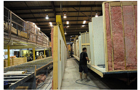
Exterior wall assemblies being set in place during manufacture
