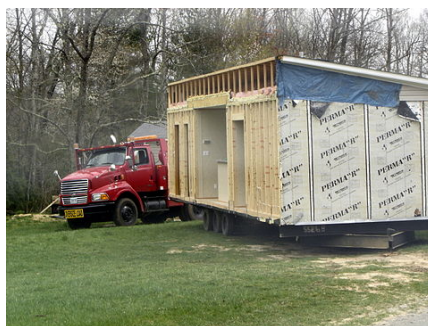
A mobile home being prepared for transport
