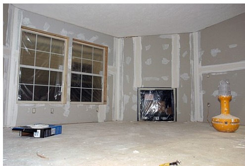
Drywall is completed.
